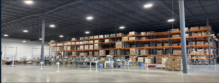
High-Bay Racked Storage
